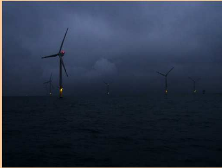
Fig. 1: Obstruction lighting on a model offshore windmill > 150 m in German waters; for smaller wind mills the "4 x obstruction lights" and "blade tip red lights" are not mandatory.
